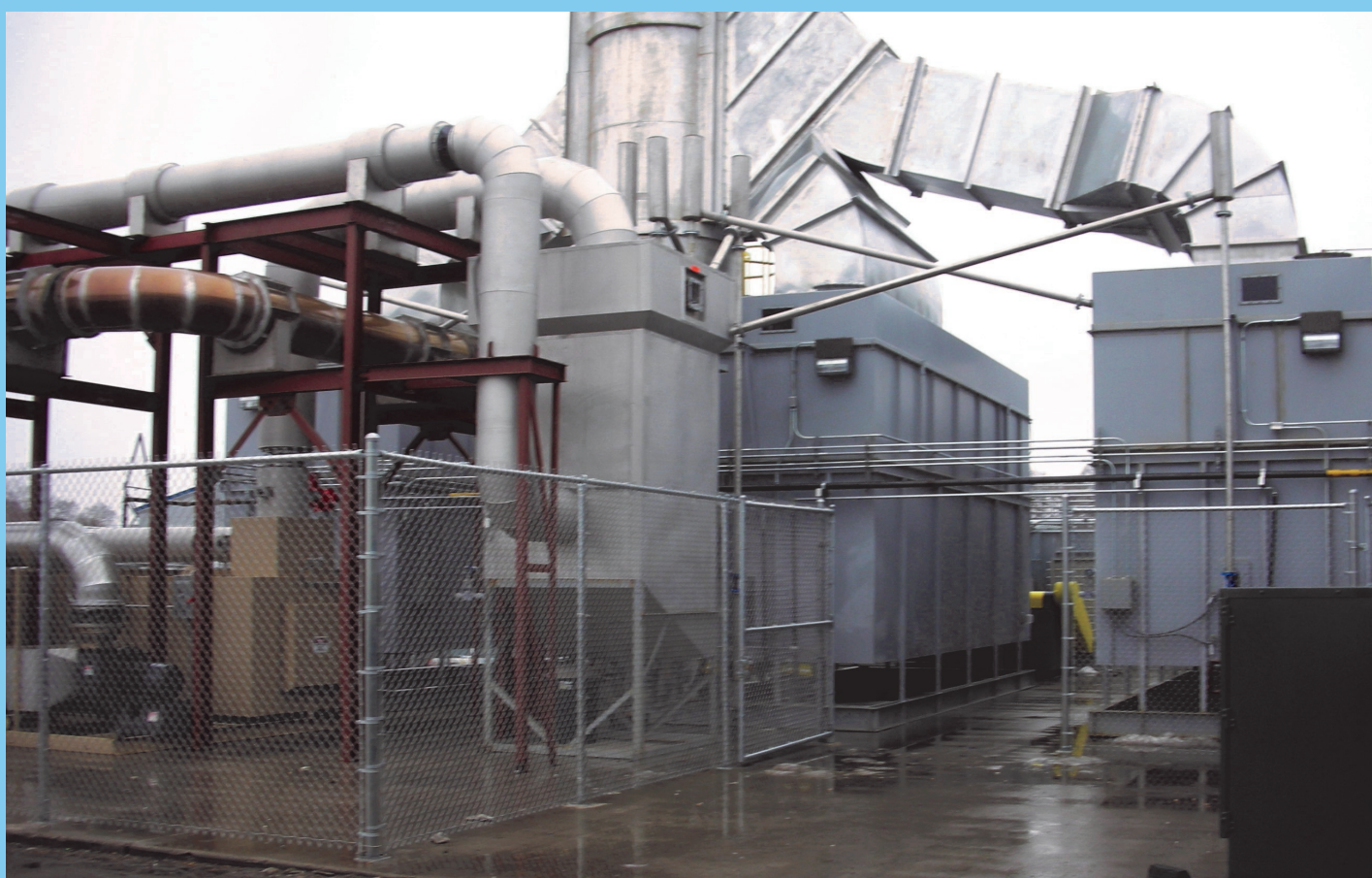
160,000 CFM Concentrator System with Oxidizer and Heat Recovery for Multi-Source Process Air Streams.—Michigan
